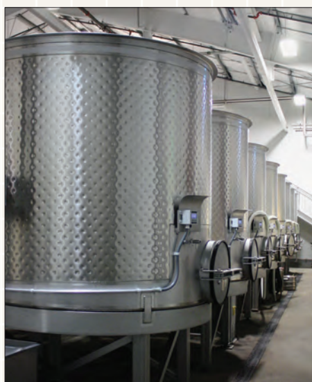
Westec’s New Tank Jackets can be built for any size tank. The 5’ total height dimpled cooling jacket provides complete temperature control.
